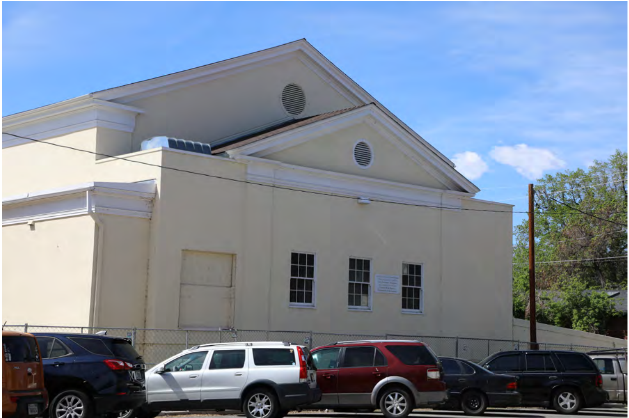
Figure 12 - Rear (north) façade, view southwest (ARG, 2024)
