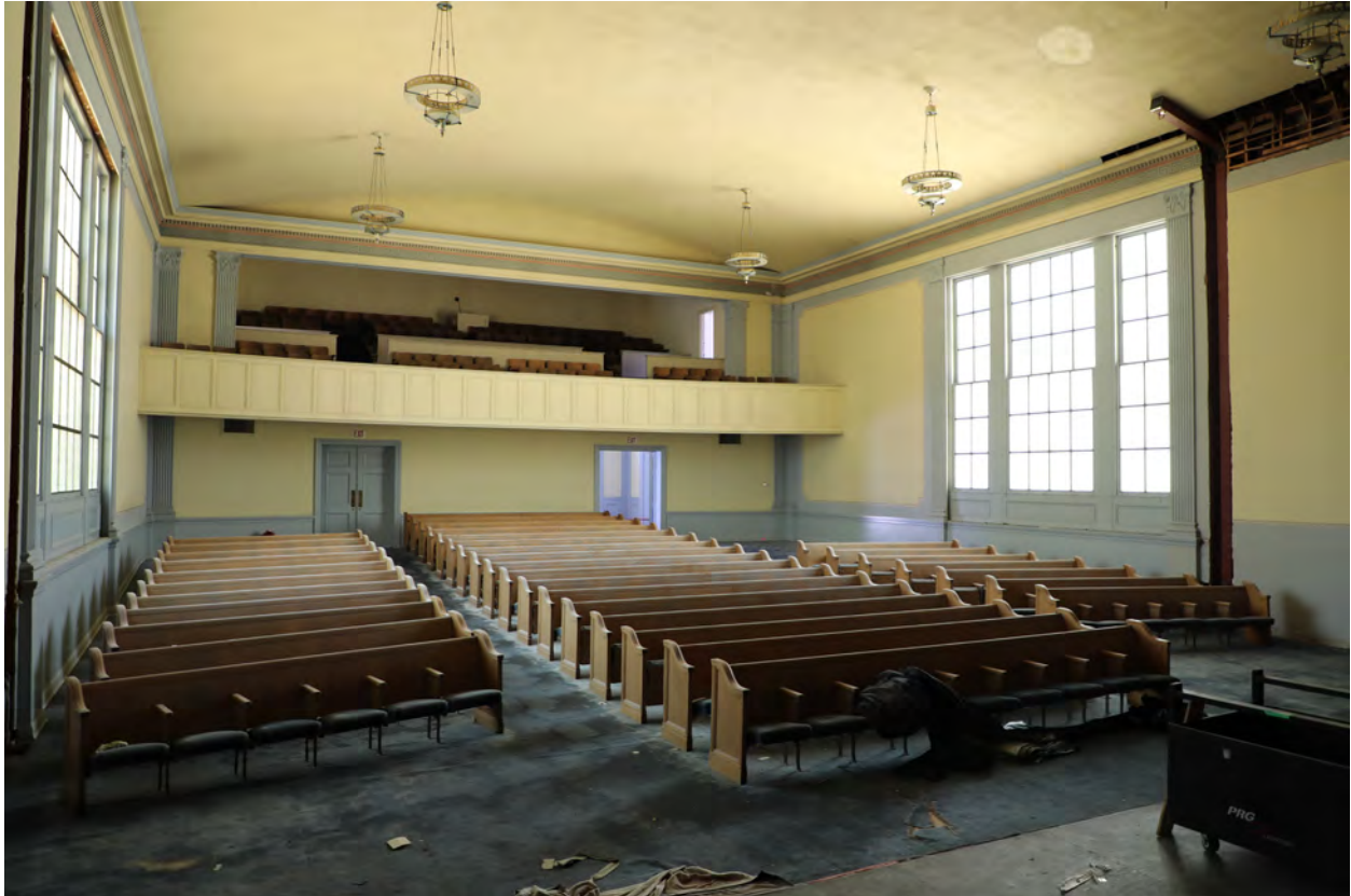
Figure 18 - Auditorium, from the stage, view southwest (ARG, 2024)
