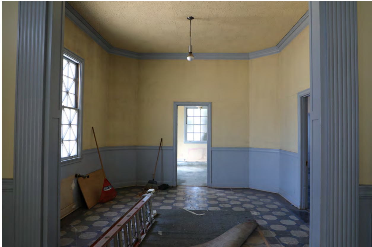
Figure 30 - West Lobby, viewed from the foyer, view west (ARG, 2024)
