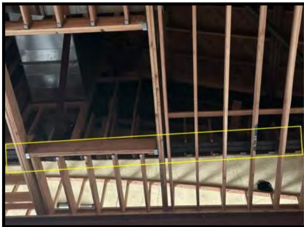
Figure 15 Exposed base of roof truss from Stage.
