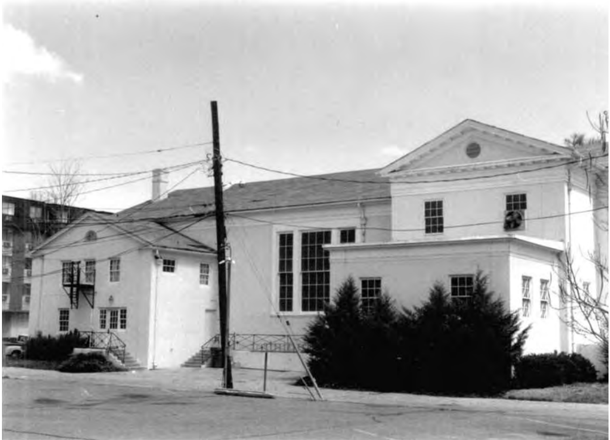
West facade, prior to 2002-2004 alterations; note rear gabled extension, entry stairs, and elevated walkway (CHECK SOURCE FOR FINAL)
