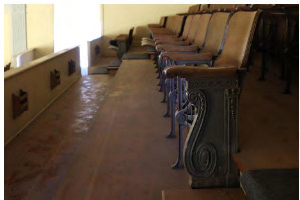
Figure 42: Original theater seating showing slight wear and tear and dust accumulation at Balcony (Room 203)
