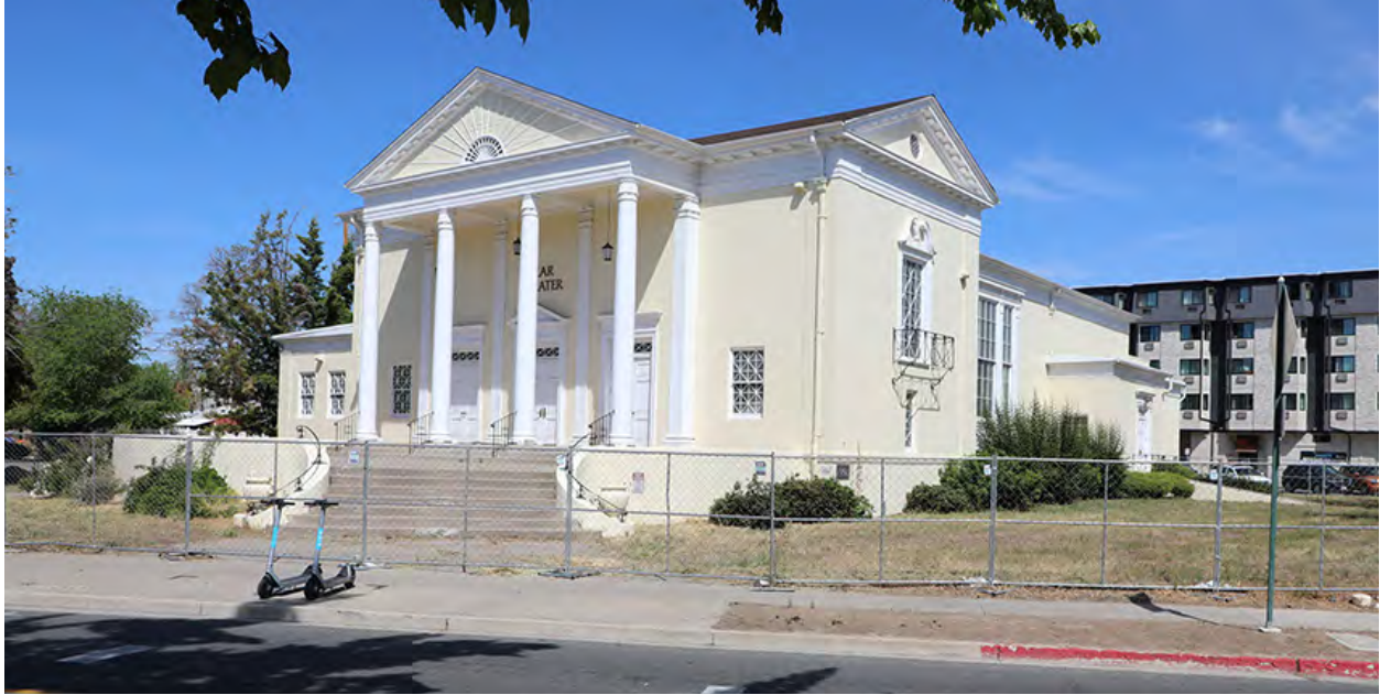
Lear Theater, primary (south) and east façades, view northwest (ARG 2024)
