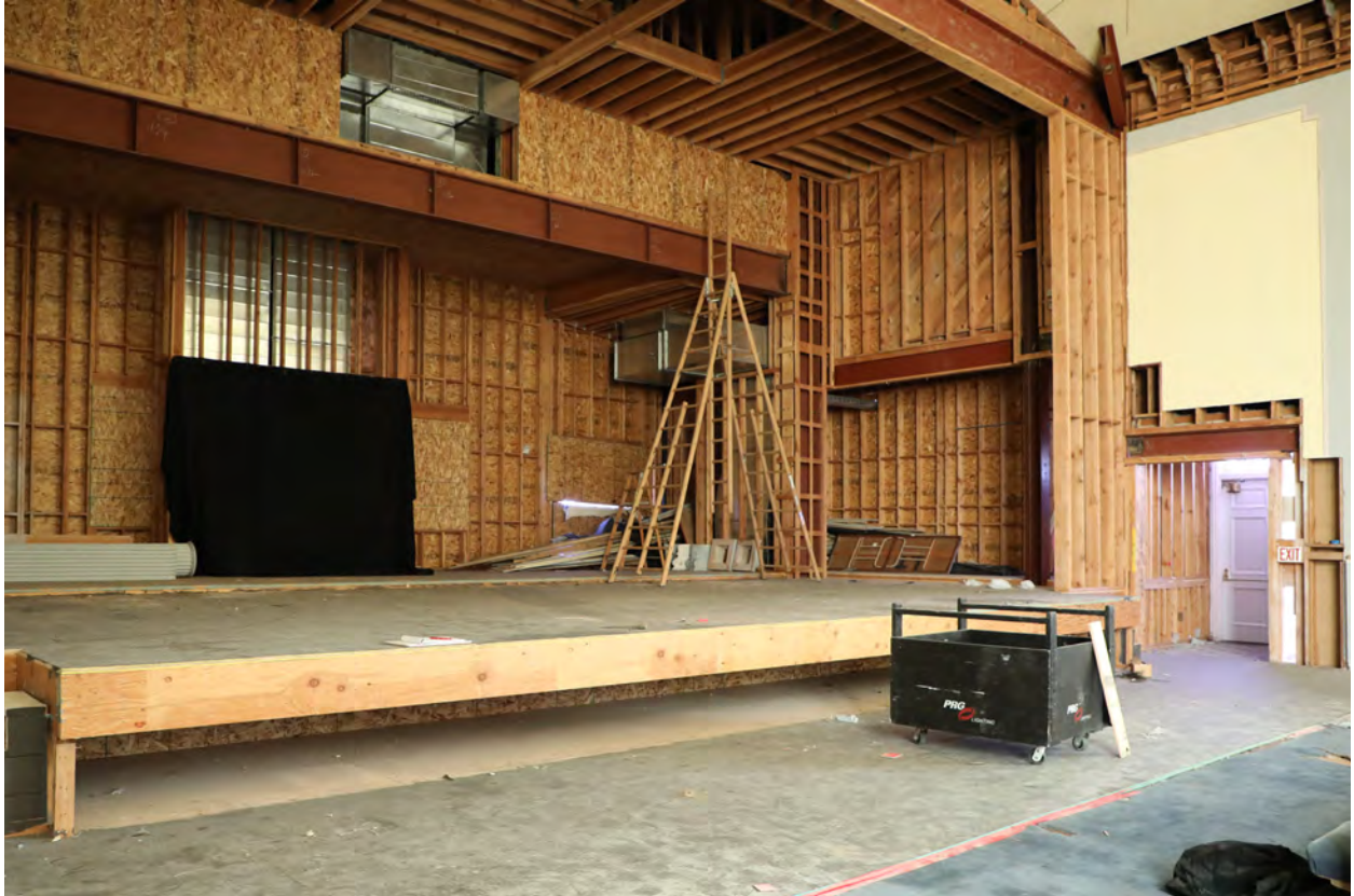
Figure 24 - Looking at stage from auditorium floor, view northeast (ARG, 2024)
