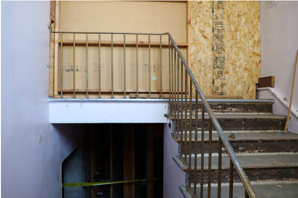
Figure 44 - North stairs from basement, looking at temporary wall, view north (ARG, 2024)
