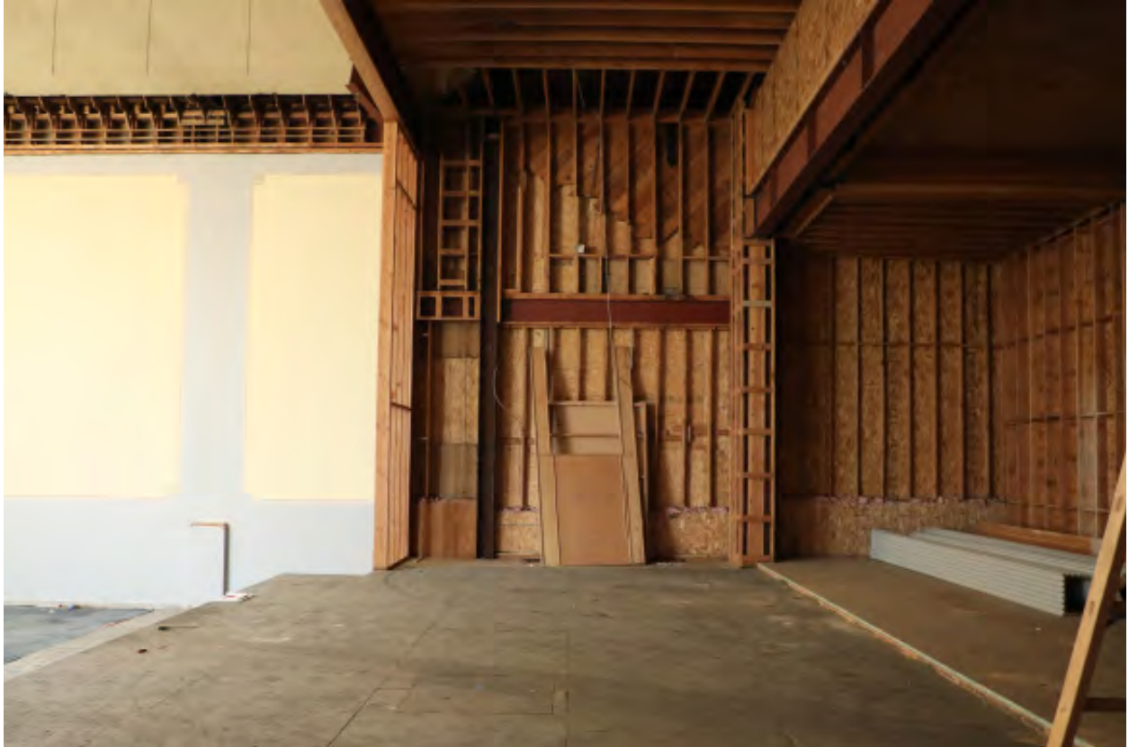
Figure 25 - looking west from east end of stage (ARG, 2024)
