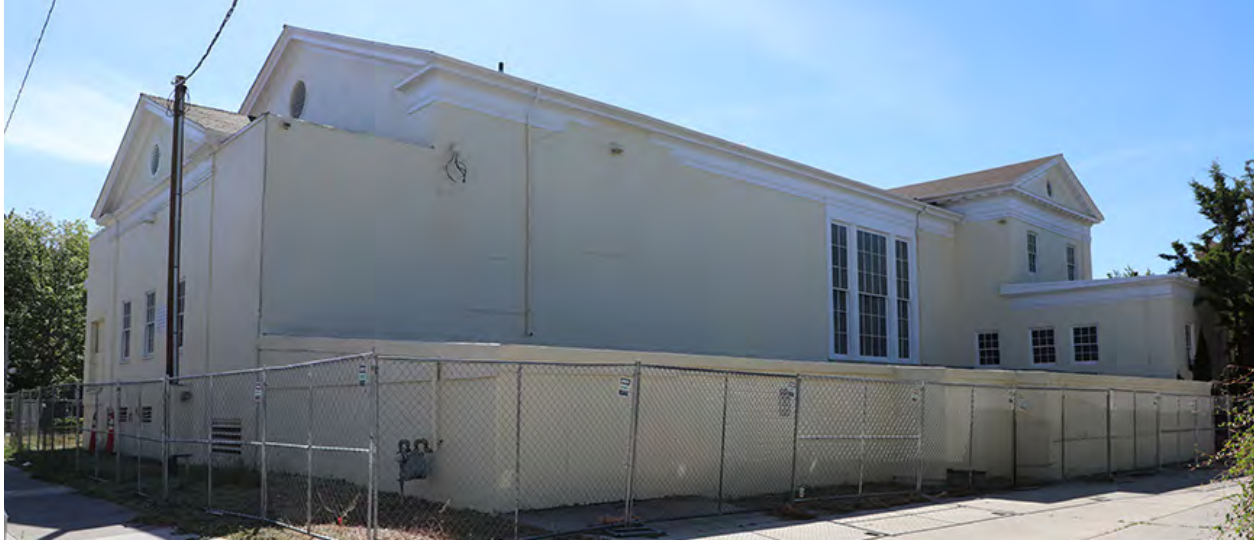
Lear Theater, rear (north) and east façades, view southeast (ARG 2024)
