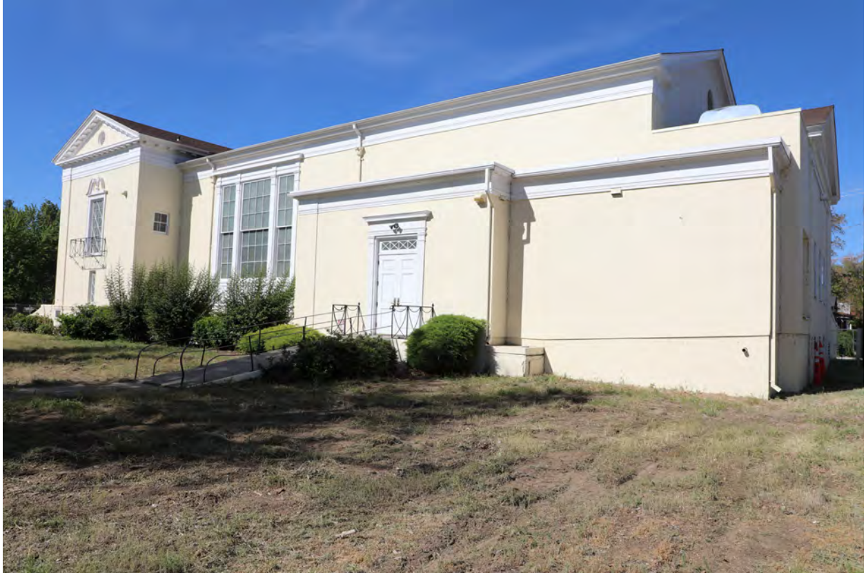
Figure 06 - East façade, view southwest (ARG, 2024)
