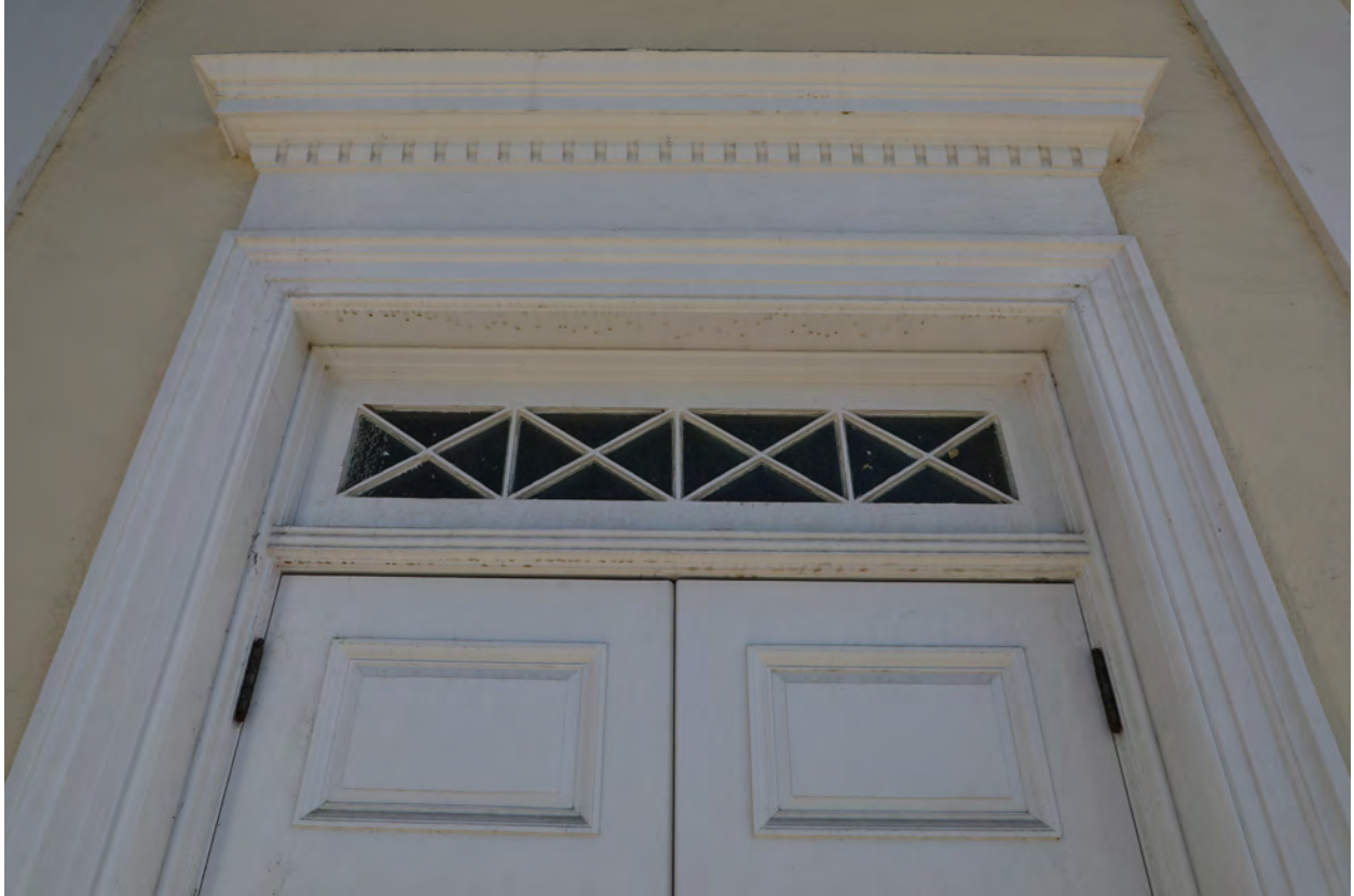
Figure 04 - Detail of entry at primary (south) façade, view north (ARG, 2024)
