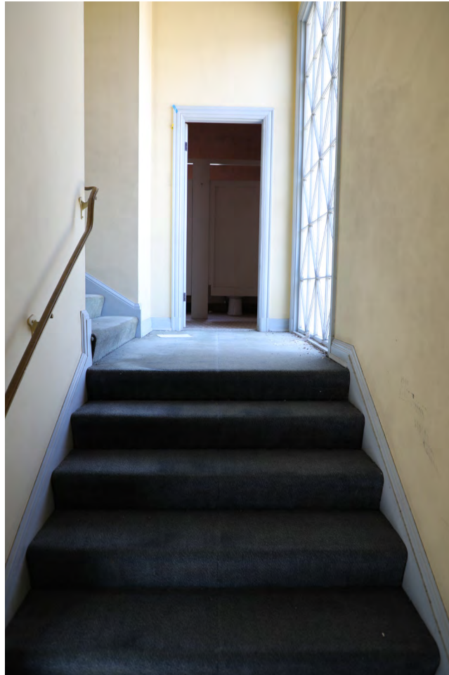
Figure 34 - Stairs to balcony looking from first landing, toward women's restroom, view north (ARG, 2024)
