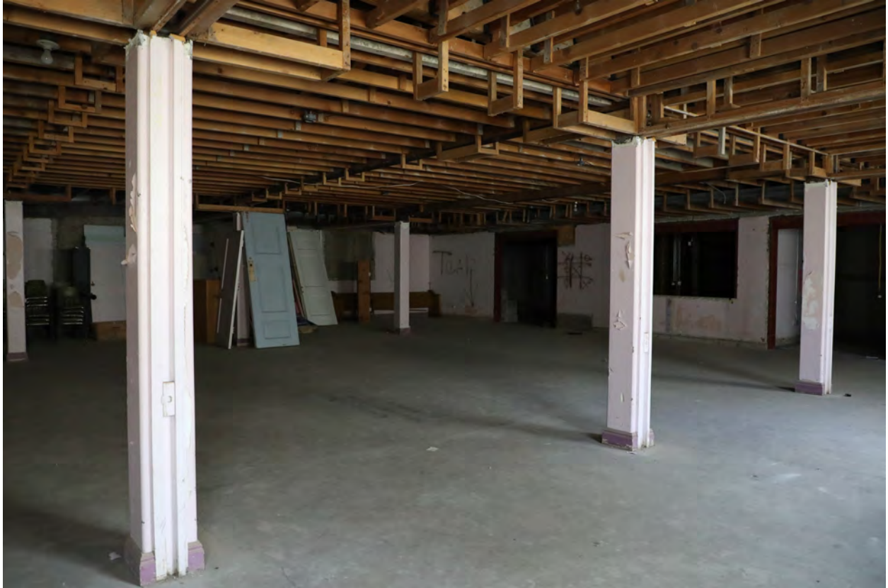
Figure 41 - Basement, cabaret theater space, view northwest (ARG, 2024)
