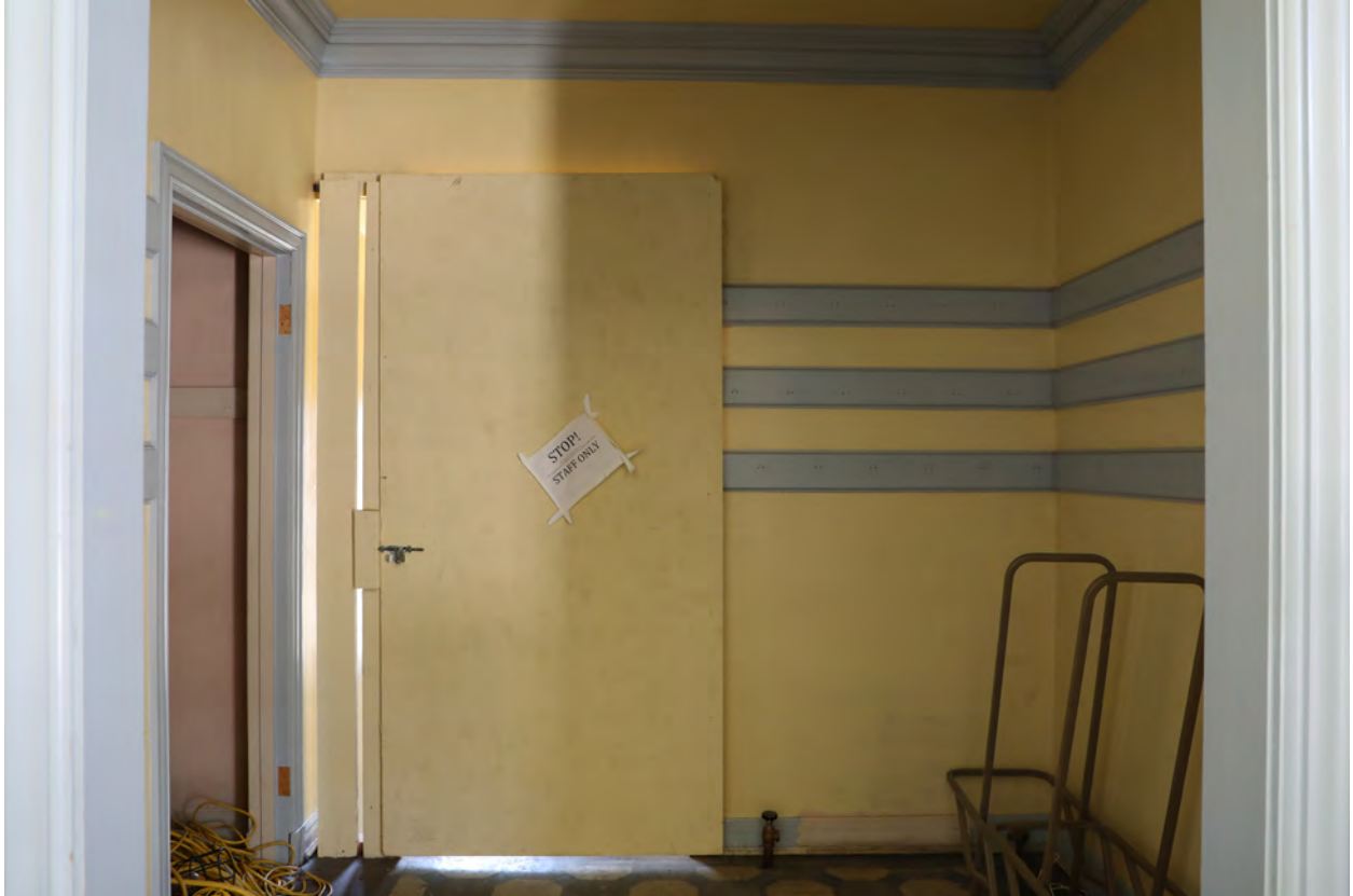
Figure 22 - Looking from foyer at temporary door in east lobby, view east (ARG, 2024)
