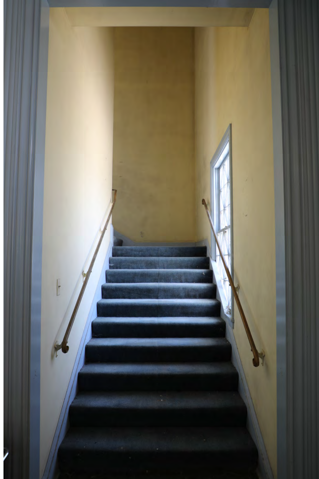
Figure 33 - Stairs to Balcony, from foyer, view east (ARG, 2024)
