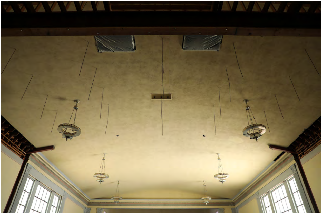
Figure 19 - Auditorium ceiling, view south (ARG, 2021)
