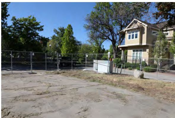
Figure 05: Extensive plant growth and spalling of the walk path at the south entry
