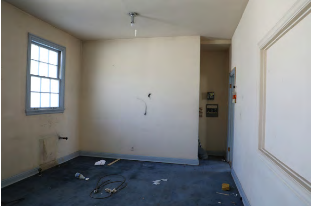
Figure 27 - Coat Room, view east (ARG 2024)
